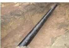
**Kebu Petro-Tape A303** is a hot-applied corrosion protection tape in accordance with DIN EN 12068 and DIN 30672, load class B at a maximum operating temperature of 30 °C.
